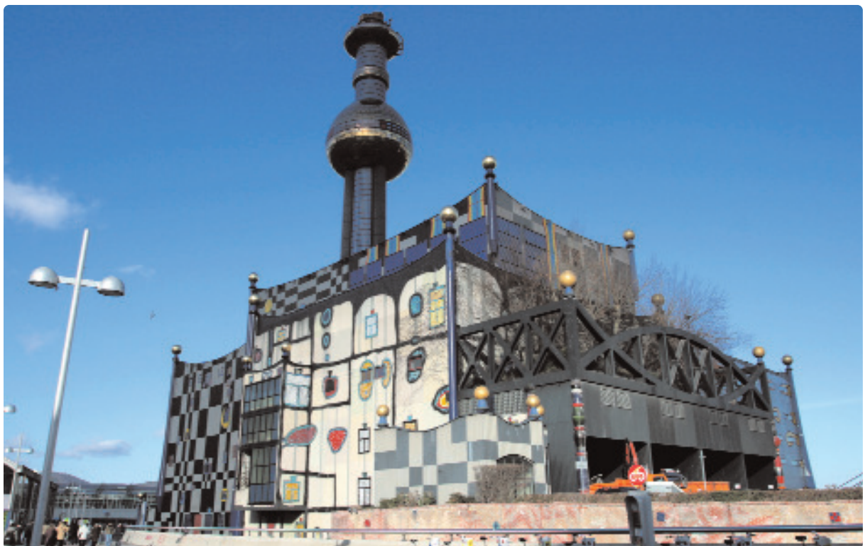
The Spittelau energy from waste and CHP facility in Vienna
